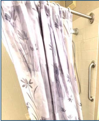
Grab bars in bathroom
