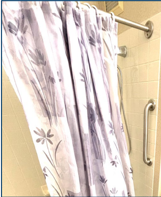
Grab bars in bathroom
