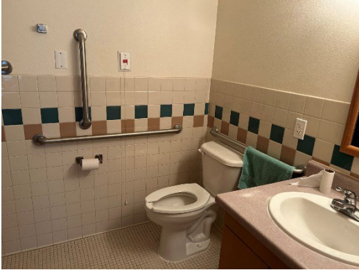
High raised toilet seat and grab bars
