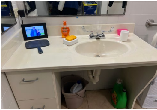
Accessible vanity in the bathroom with room for a wheelchair
