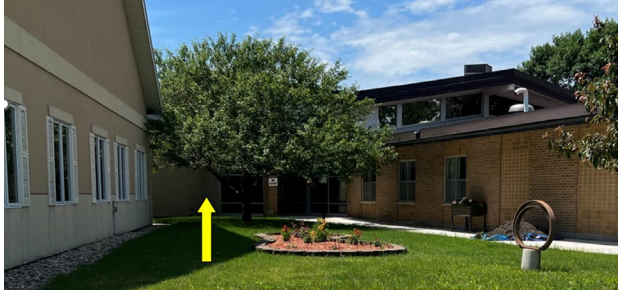
Yellow arrow indicating the hallway connecting the two settings.
