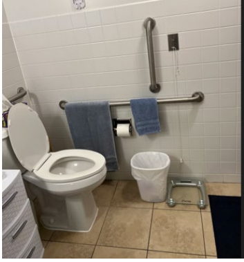
Bathroom with grab bars
