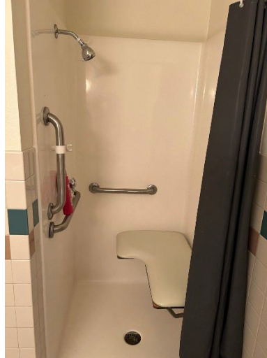
Grab bars and shower seat in residents bathroom
