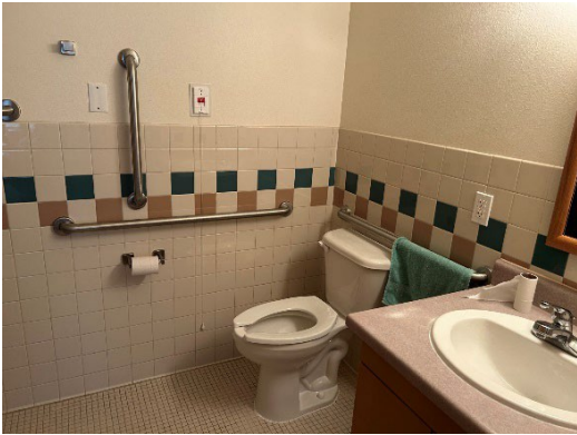
High raised toilet seat and grab bars
