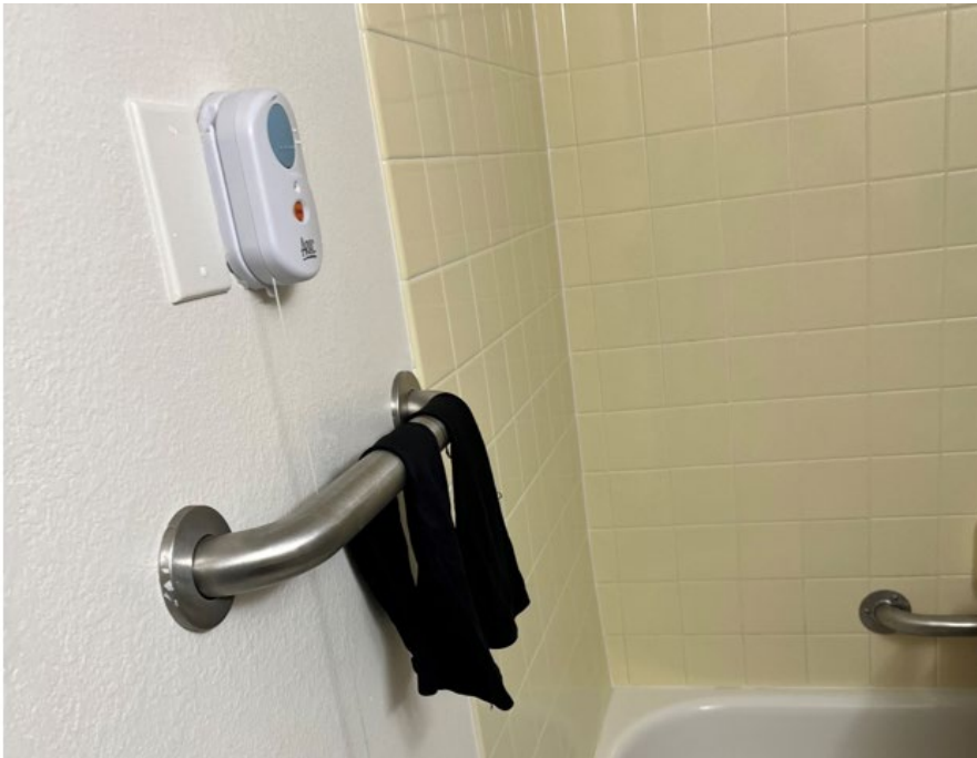
Grab bars in the resident's bathroom
