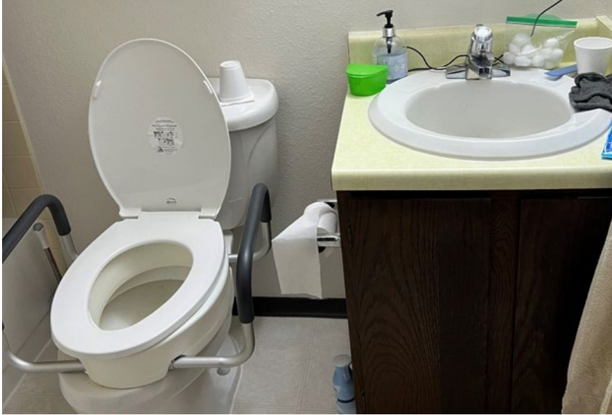
Resident's bathroom with bars for accessibility
