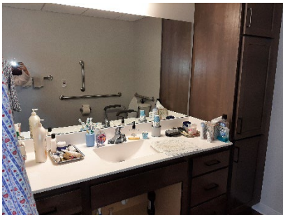
Resident's bathroom area with accessible sink, grab bars and toilet riser
