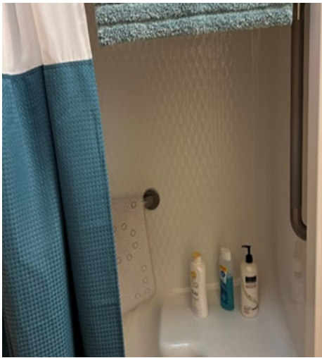
Bathroom with grab bars for accessibility
