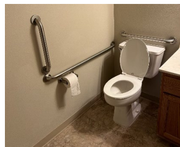
A picture of a bathroom with accessibility features such as grab bars
